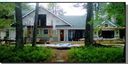
sense of enclosure at the deck, but it also adds a shading element to the windows of the Great Room and along with deeper overhangs at the Dining area, it reduces heat gain and lowers energy costs related to
